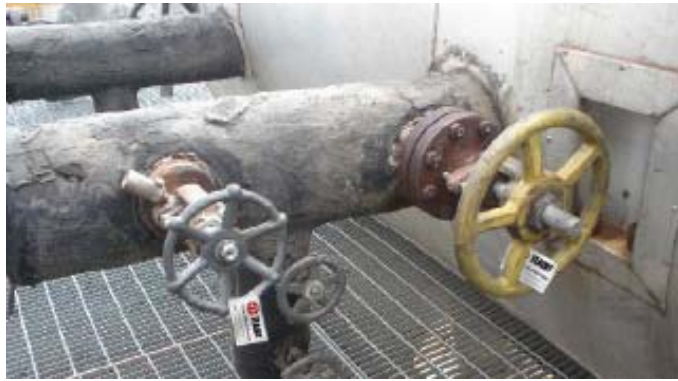
FIGURE 15 – LEAK-FREE VALVES AFTER S_s WAS APPLIED
