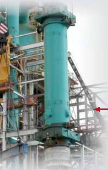
Gimbal Cold-wall Expansion Joint - ID 64 in
