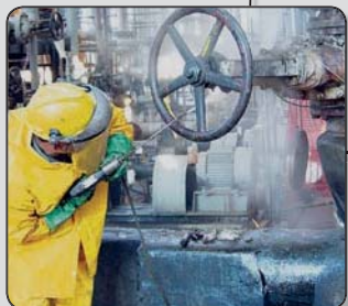
Valve Stem Packing Extraction
