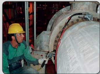
Controlled Torque Gasket Installation
