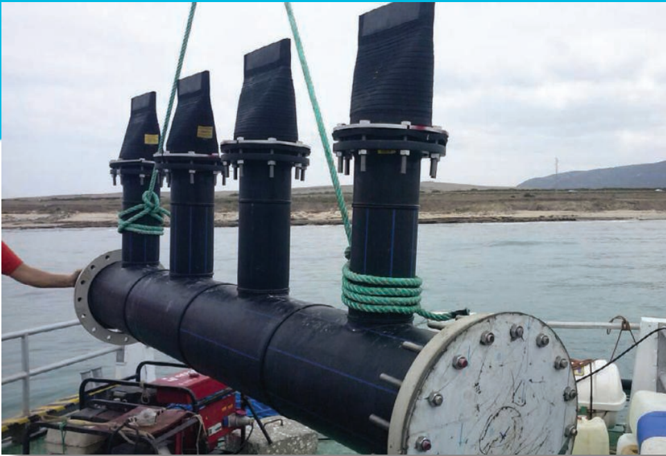
Detail of the ProFlex™ Flanged Rubber Check Valve; Style 710
