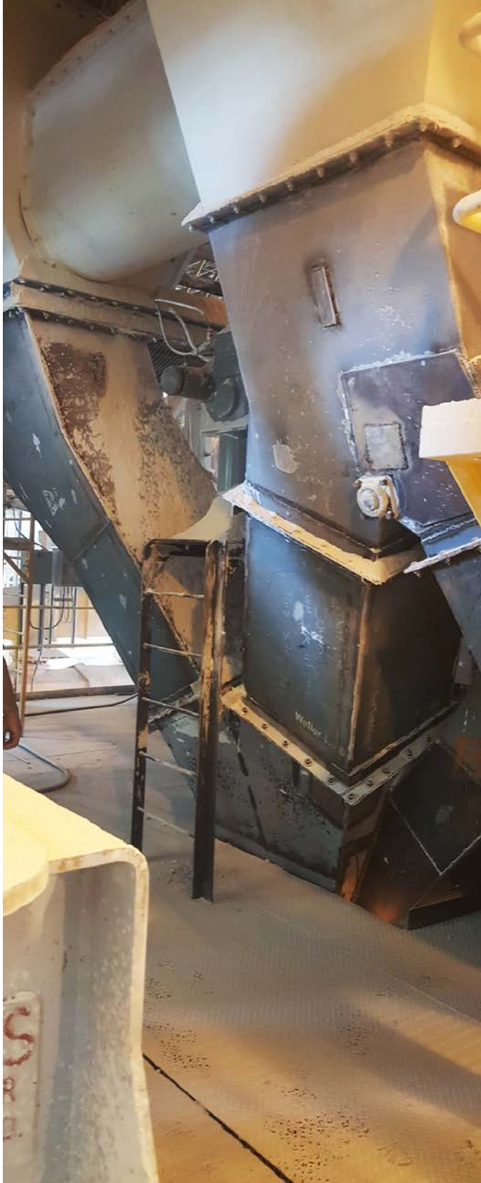
Transfer Chutes Before
