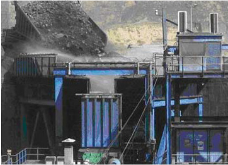
Truck Unloading Hopper
