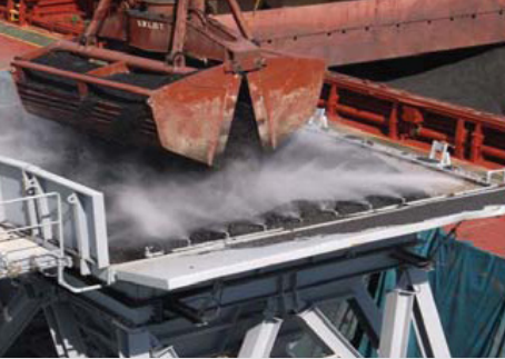
Ship Unloading Hopper
